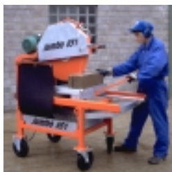
Large block being cut.
