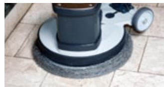
Vitrification of marble floors
