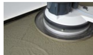
Smoothing of concrete
