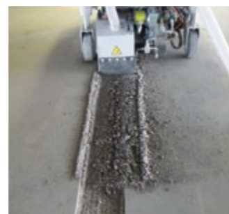
Oscillating milling = low operation weight
